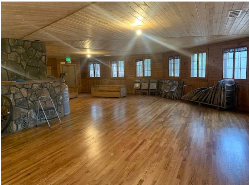
Roundhouse new floor and ceiling
