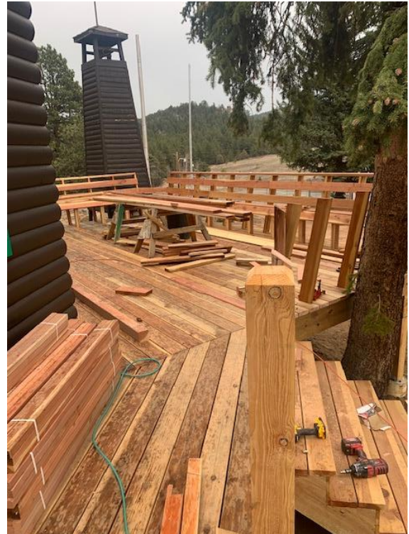
New deck is nearly completed
